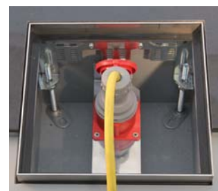
CEE socket with straight connector
